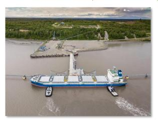
Partnered with Matanuska-Sustina Borough to demonstrate how predictable output from tidal devices can provide baseload power to the port's cathodic protection systems for corrosion prevention.
