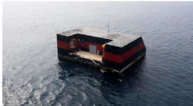
View of the Yongsoo Wave Power Plant © KRISO
