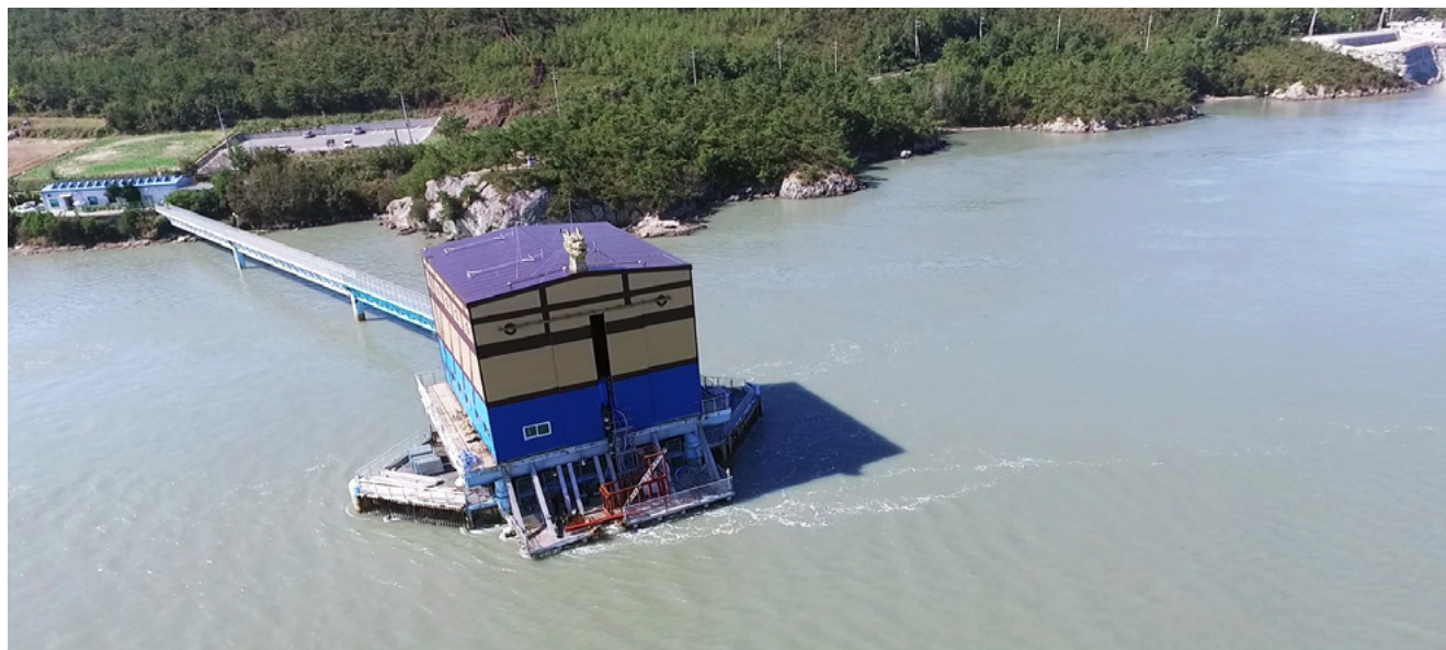
Uldolmok Tidal Power Station © KIOST
