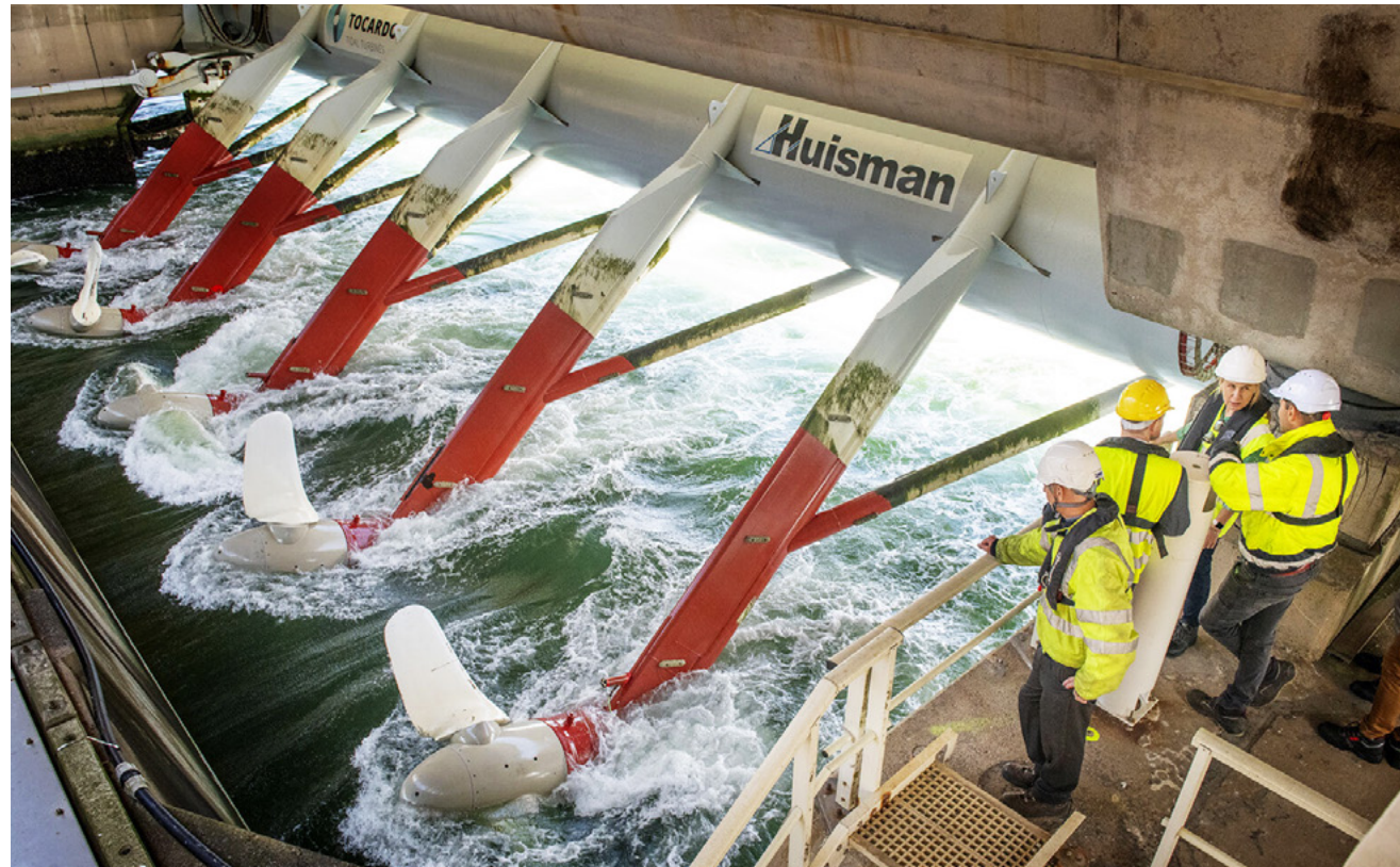
Tocado's Oosterschelde Tidal Power Plant © Tocardo
