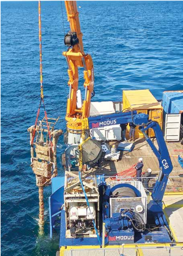
Connexion upgrade at Paimpol-Brehat tidal site: former wet-mate replaced by dry-mate
