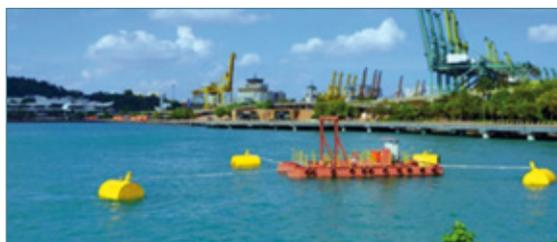
*Barge based floating tidal system*
